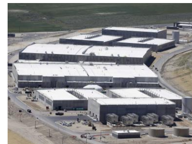
Utah data center [1]
